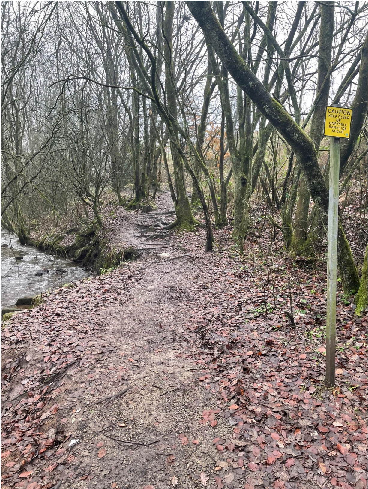
Photograph 15: Shows the route of footpath 26 going east from path routes from Ashbrook Road and sign which states “Caution Keep Clear of unstable bank side ahead”
